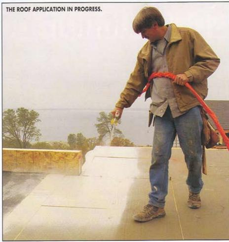
additional fire protection." MOS provides adhesive qualities, fire protection and a hard surface where it is most needed. When used in combination with specially developed SBS membranes, the MOS system provides resistance to puncture, wind uplift, and traffic.
